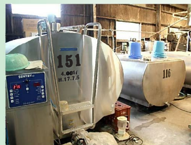
Milk coolers to cool tanks
