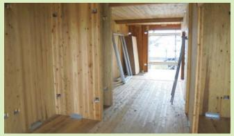
Housing complex (under construction)\*CLT panel construction method
